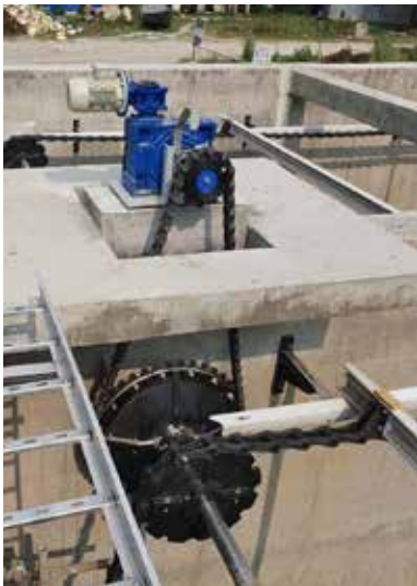
Driven sprocket, Head sprocket, Drive chain, and Drive system by helical bevel gear motor and reducer.
