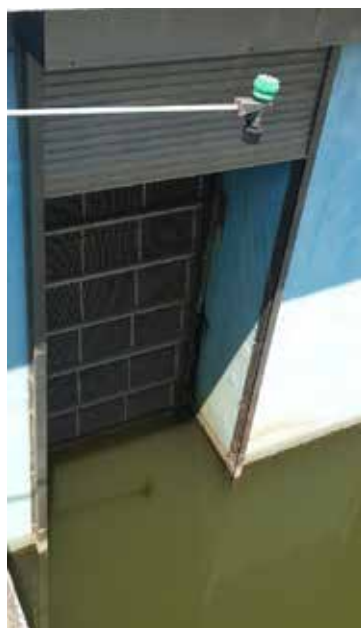
4mm mesh opening of mesh screen is made of stainless steel 304, 316.
