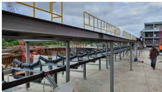
Horizontal belt conveyor, 51m installed together with 4 rotary screens and platform in apumping station, Bangkok, Thailand 2019.
